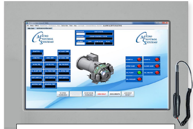
COMPRESSOR OVERVIEW SCREEN
